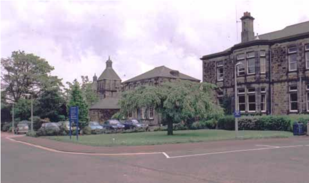
● Driveway to the north of the Dyson complex
