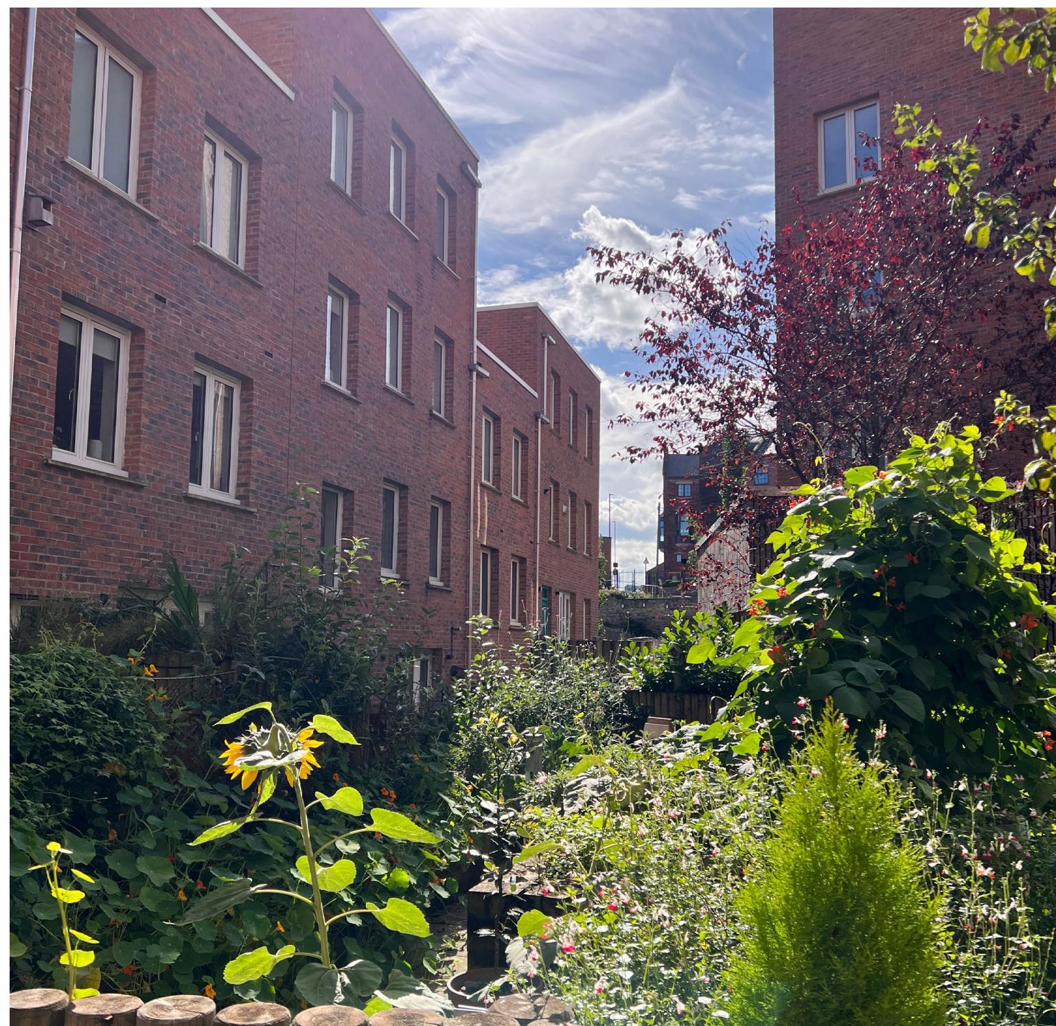
The Malings, Ouseburn - has shared bin storage areas for residents in undercroft areas with a central communal recycling facility.
