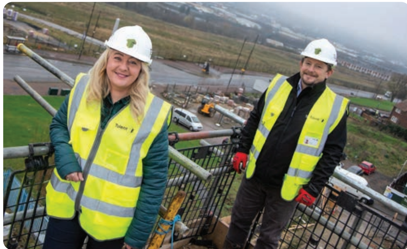
Councillor Linda Hobson, Cabinet Member for Housing and Ian Avis, Regional Construction Manager at Tolent, admire the views across the Tyne from the roof of Addison Court
