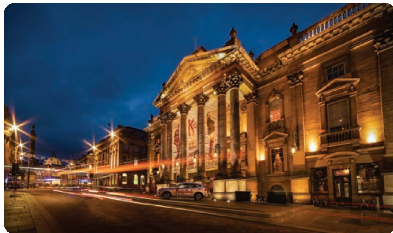
The Theatre Royal, which is one of 32 buildings that will benefit from our successful bid for £27.25 million in funding for low carbon upgrades
