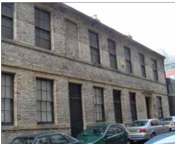
• 20 South Street - grade II* listed, former offices of Robert Stephenson and Company.
