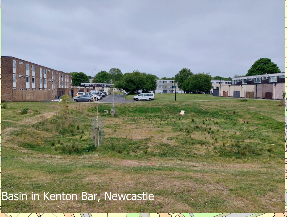
Rain garden. (C) Meristem Design Ltd 2026
