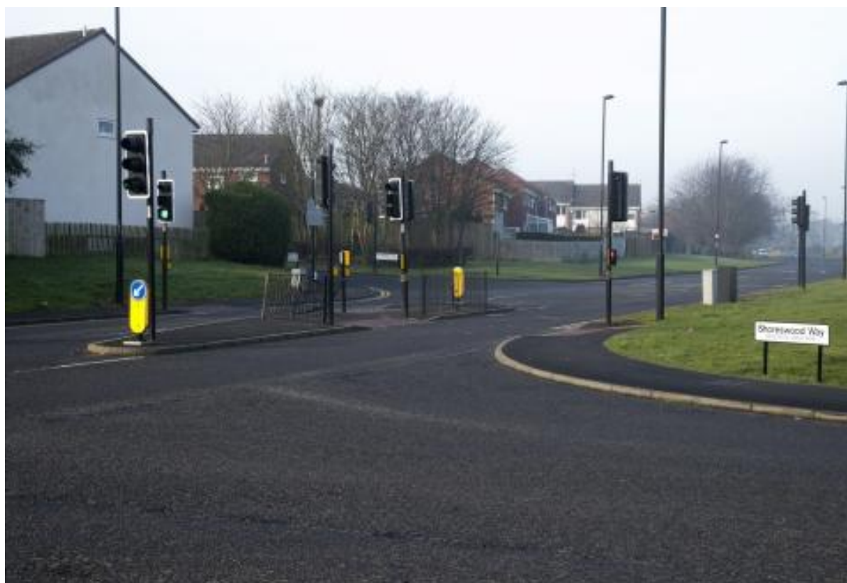
Figure 1: Kingston Park Road Carriageway Widening
