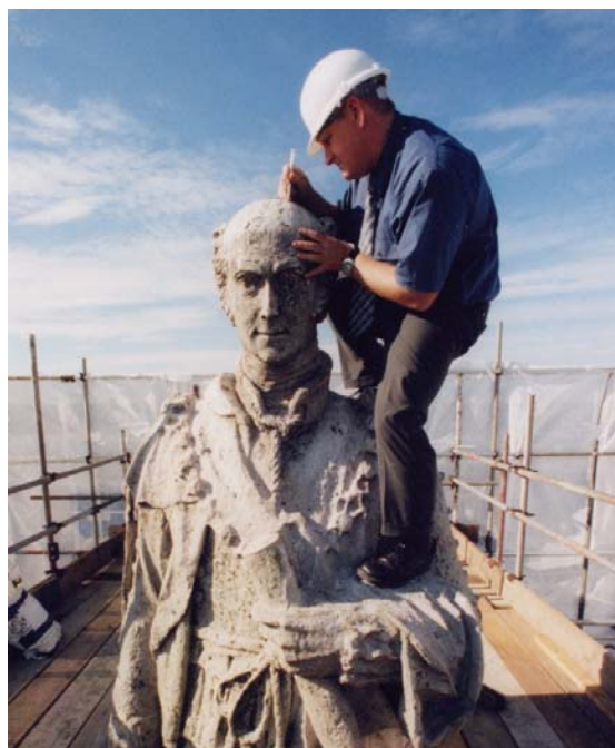
Above: Stonemason Michael Moody repairing Earl Grey's head on the Monument.
